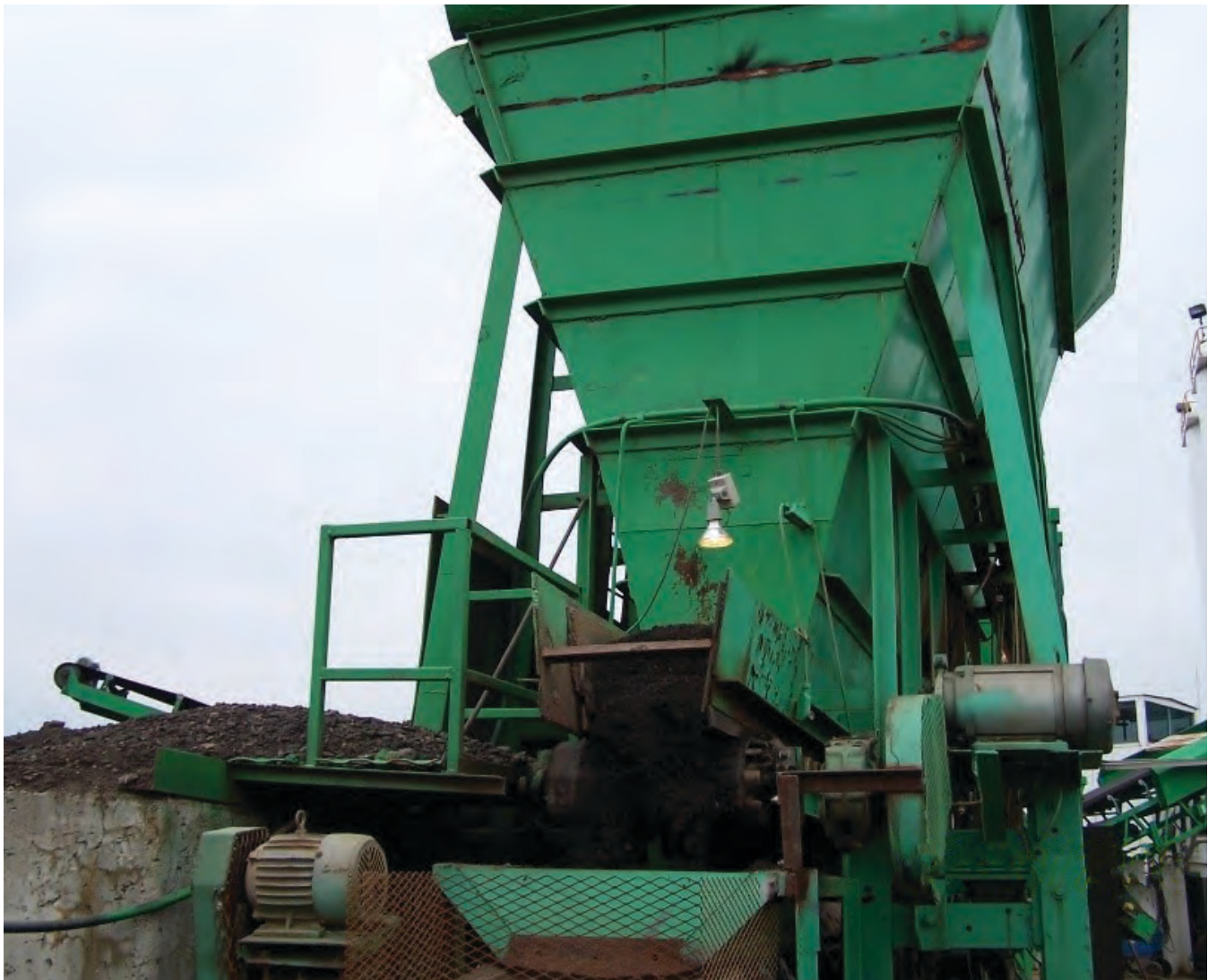
Figure 4-1. Steep-sided RAP cold feed bin.
