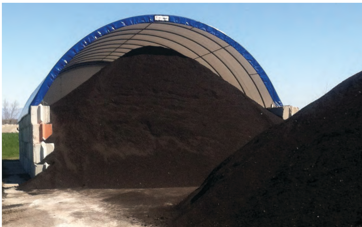
Figure 5-2. Covered RAS stockpile.
