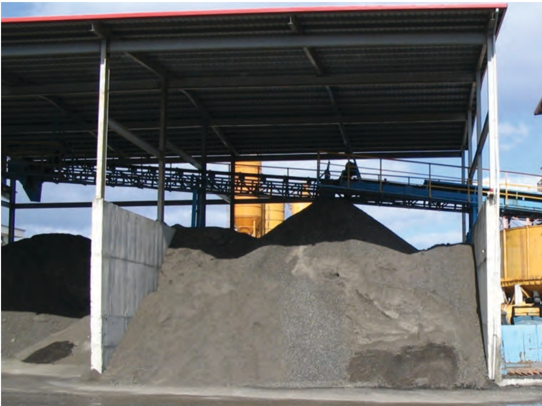
Figure 2-8. Covered stockpile to minimize moisture in RAP.
