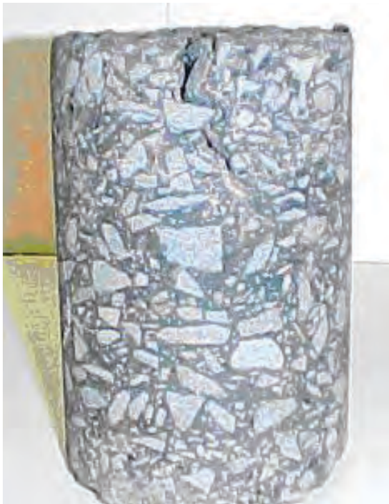
Figure 1-2. Roadway cores showing distressed layers: top-down cracking on top; stripping damage on the bottom.
